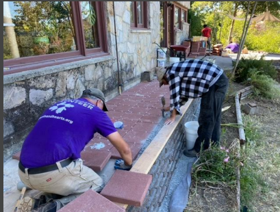
Pavers replaced old decking in Zone Zero
