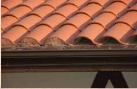
Only 1/2 of the tiles shown in this image have bird-stops installed. Embers may ignite debris beneath the exposed tiles.
