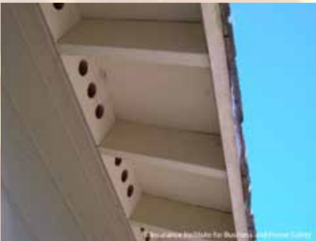
Open-eaves and eave-vents are particularly vulnerable to flames and embers.
